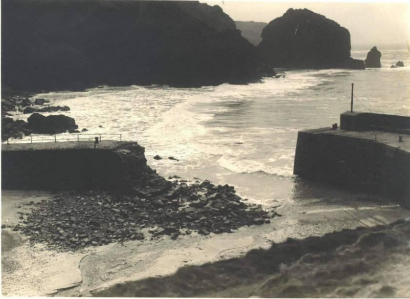
Damage to Mullion Harbour's southern breakwater, 1946 (National Trust).
